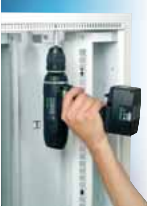
1. Position the distribution cabinet in the wall cut-out such that its front surface is flush with the wall, and then fasten it to a supporting frame installed around the cabinet inside the wall cavity.
