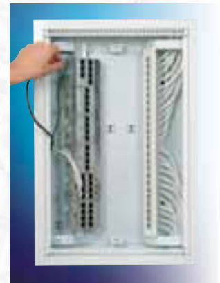
8. Connect the incoming cables/wires to the active modules. Connect the 12V DC power supply to the data and TV amplifier modules.
